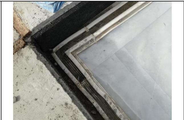
Separate Casting of PVC Waterstop
